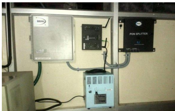
Fig. 3.5.22 ONT Connectivity with Splitter and CCU- Wall Mount 1
