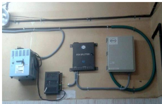
Fig. 3.5.22 ONT Connectivity with Splitter and CCU - Wall mount 2
