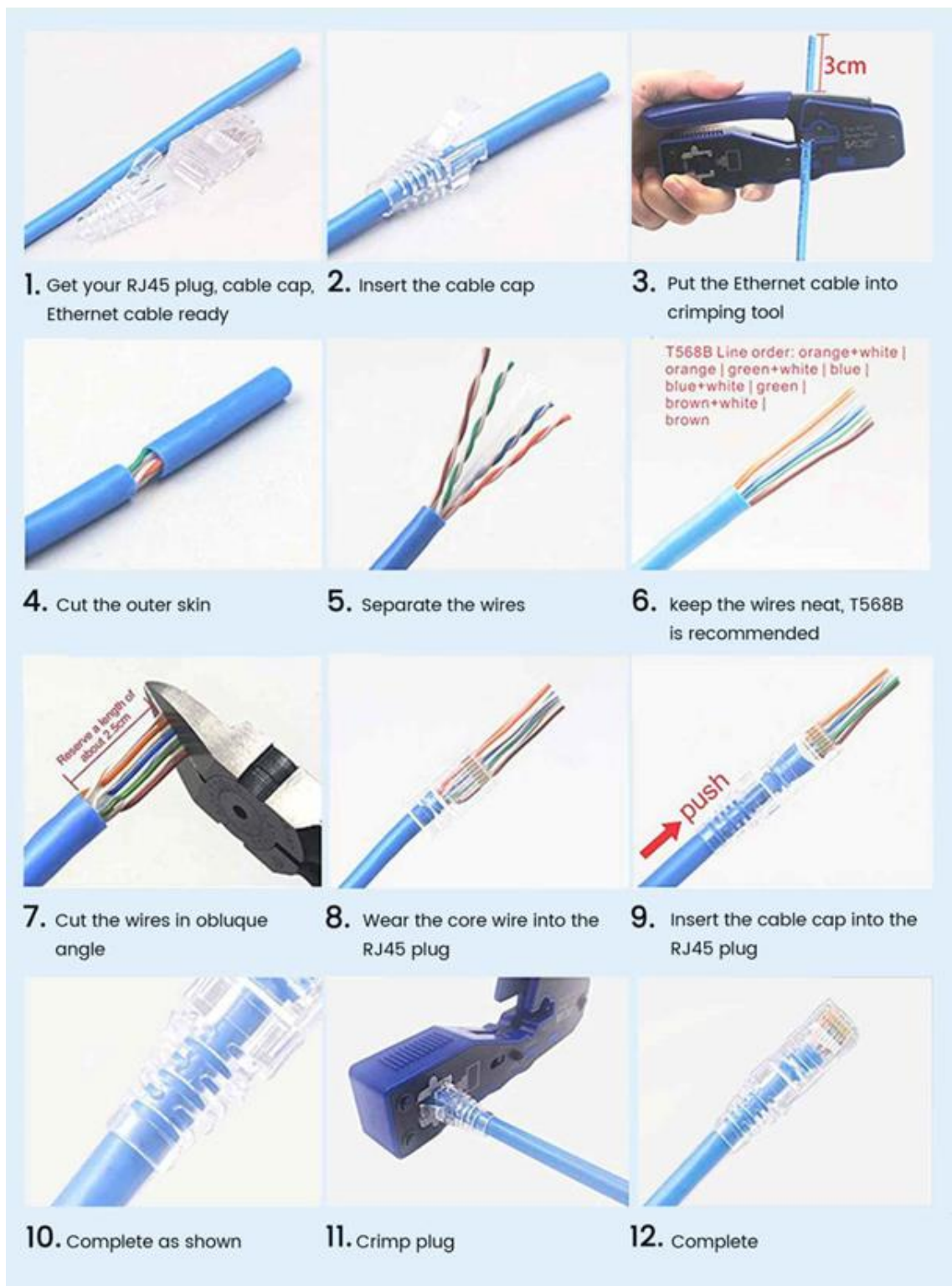
Fig 2.2.3 Steps for Crimping
