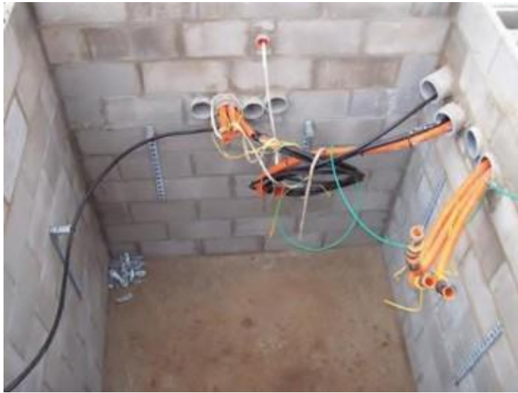
Fig. 6.2.10: Pulling Fiber through Conduits
