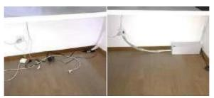
Fig. 2.5.17: Safe and unsafe power cable arrangement
