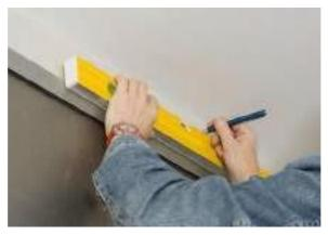
Fig. 2.6.2: Marking the surface
