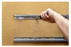
Fig. 2.6.7: Mounting camera bracket on wall
