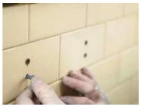
Fig. 2.6.4: Wall anchors in drilled holes
