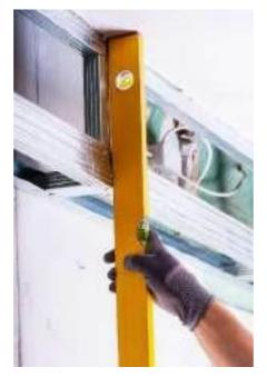
Fig. 2.6.1: Checking the surface level
