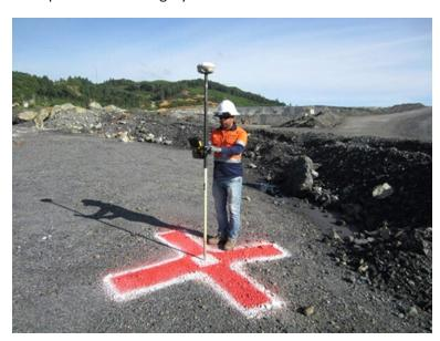
Fig.4.1.9 setting ground control points
