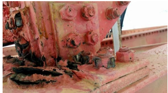
Fig. 3.1.1: Corrosion in Telecom Tower
