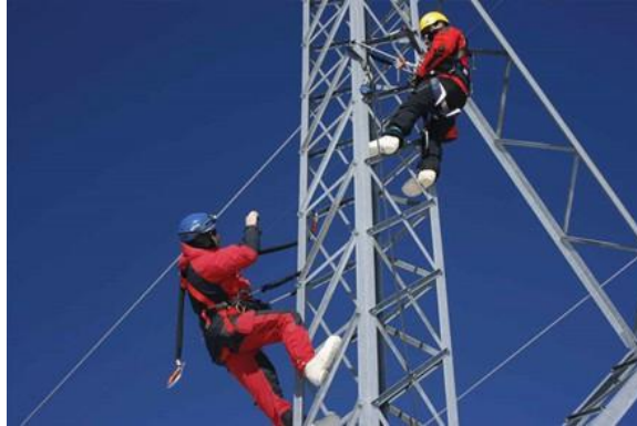
Fig. 4.1.10: Safety Cable Climb / Fall Protect System illustration
