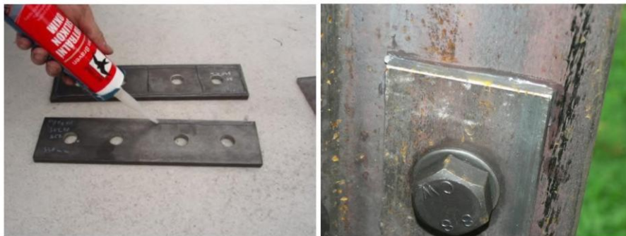
Fig. 3.1.2: Corrosion Resistant Sealants for Joints
