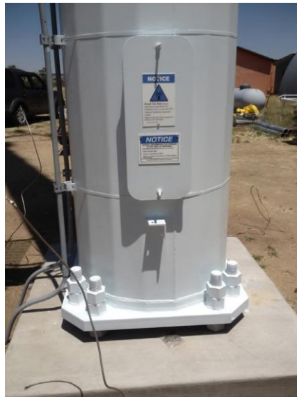
Fig. 2.2.11: Base of a Monopole Tower
