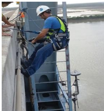
Fig. 4.1.11: Tower climbing using two or more lanyard
