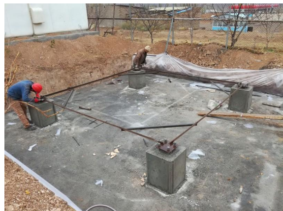
Fig. 2.2.10: Foundation of a Telecom Tower
