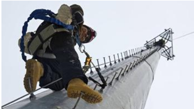
Fig. 2.1.9: Fall Protection System while Climbing Monopole
