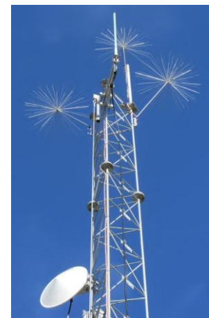
Fig. 2.2.18: Lightning Arrestor
