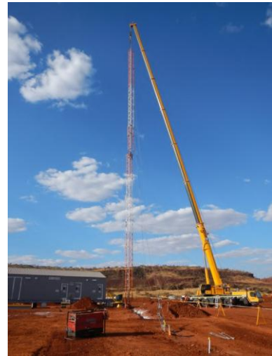
Fig. 2.2.14: Construction of Guyed Tower
