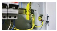
Fig. 3.3.7: Grounding and Bonding
