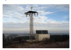
Fig. 3.1.3: Power Supply Systems for Telecom Tower
