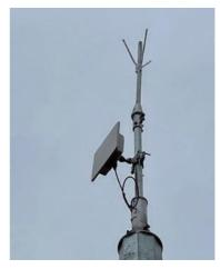
Fig. 3.1.5: Lightning arrester
