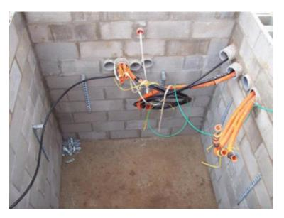
Fig. 5.2.10: Pulling Fiber through Conducts
