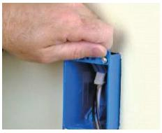
• Connect the electrical fixture to the electrical box using wire connectors.
