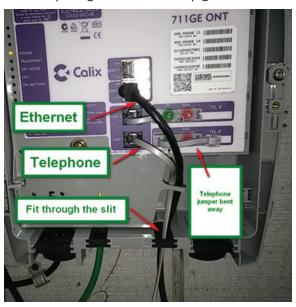
Fig. 5.3.2: Optical Network Terminal (ONT)
