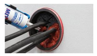
Fig. 1.3.16: Duct Sealing
