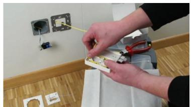
Fig. 2.2.13: Securing Extra Cable at the Termination Point
