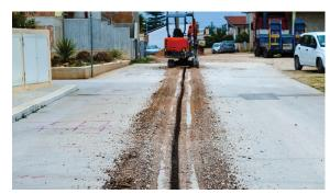
Fig. 4.3.2: Micro-trenching for optical fibre laying
