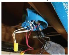
Secure the electrical fixture to the electrical box using screws.
