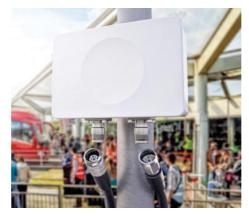
Fig. 3.1.5: Connection of RF cable
