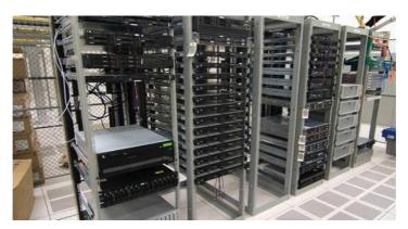
Fig. 2.2.15: Placing heavy equipment at the bottom of racks
