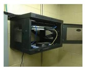
Fig. 2.1.2 Wall mounted rack
