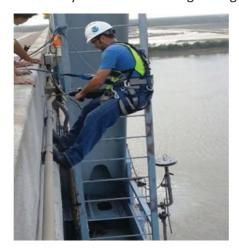
Fig. 4.1.11: Tower climbing using two or more lanyard
