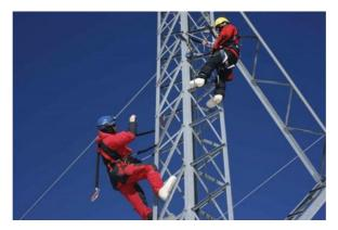
Fig. 4.1.10: Safety Cable Climb / Fall Protect System illustration
