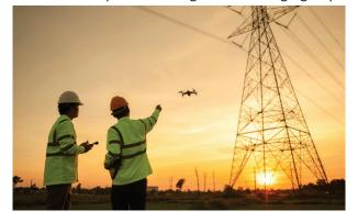
Fig. 5.2.1: Inspecting transmission tower using drone
