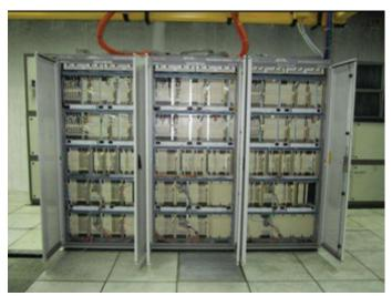
Fig. 1.2.6: Mobile Switching Centre Room Equipment
