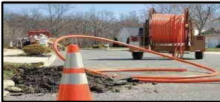
2.1.1 : A site visit in progress
