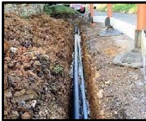
2.4.11.1 : Ducting process
