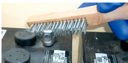
Fig. 2.5.13 Cleaning of Batteries
