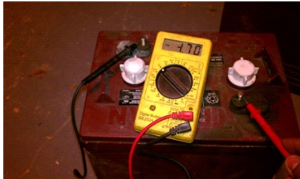
Fig. 2.5.9 Checking Battery Voltage
