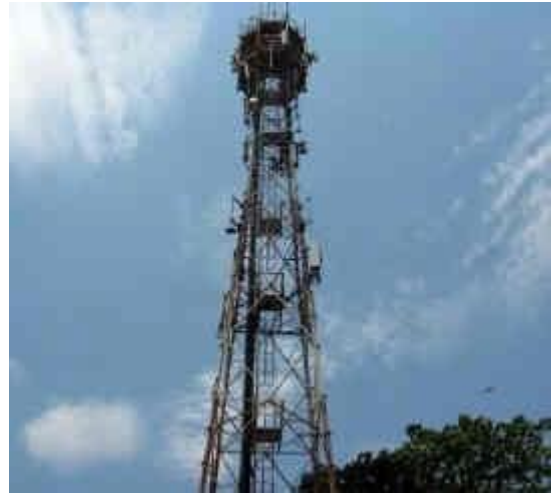
Fig. 1.2.2(ii): A telecom tower
