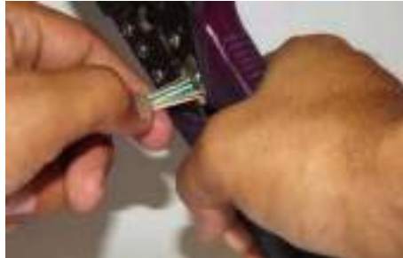
Fig. 2.3.17: Trimming of wires
