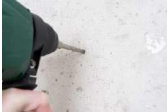
Fig. 2.5.7: Drilling on wall
