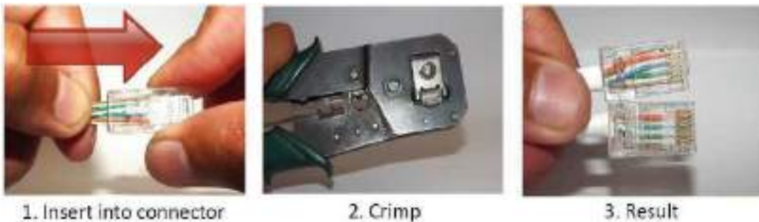
Fig. 2.3.18: Crimping the connector
