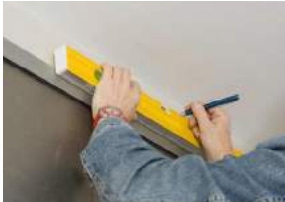
Fig. 2.6.2: Marking the surface
