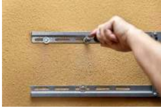
Fig. 2.6.7: Mounting camera bracket on wall
