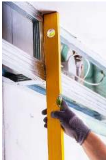
Fig. 2.6.1: Checking the surface level
