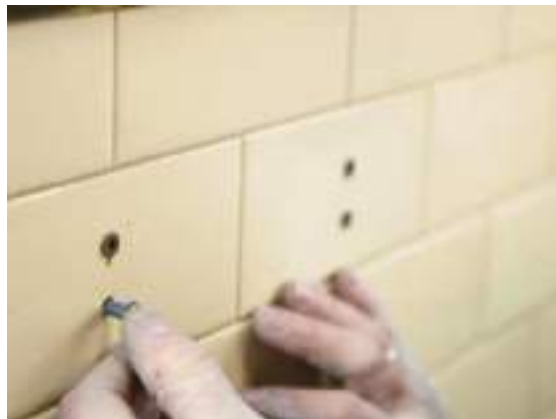
Fig. 2.6.4: Wall anchors in drilled holes
