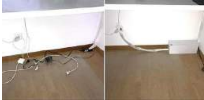
Fig. 2.5.17: Safe and unsafe power cable arrangement
